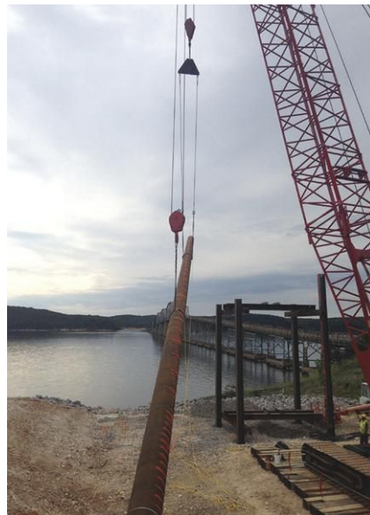
A two-lane truss bridge was replaced with a four-lane bridge designed with pipe piles with low diameter-to-thickness ratios for the seismic area in Kentucky.
