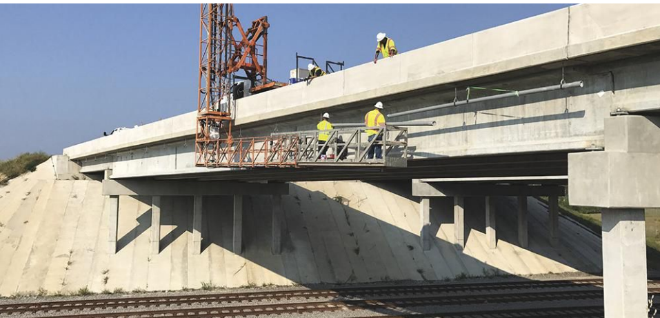
Aptus was called in for a change order and installed 8,000 ft of 4-in. multicell pipe on the I-140 Wilmington Bypass that crosses Cape Fear River.
