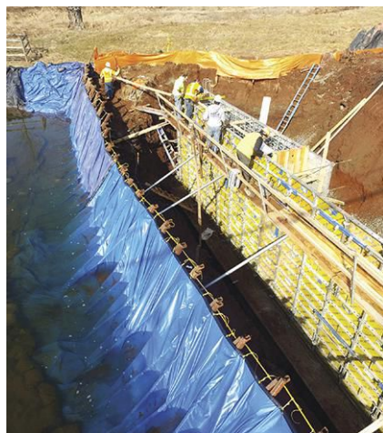
The South Branch Road Bridge was replaced with the help of a cofferdam, which kept the area dry during construction.
