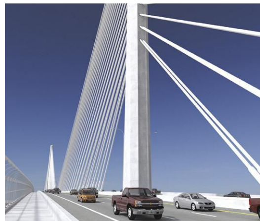
The concrete bridge design for Harbor Bridge provides corrosion resistance and preventive maintenance, enabling the bridge to last more than 170 years.
