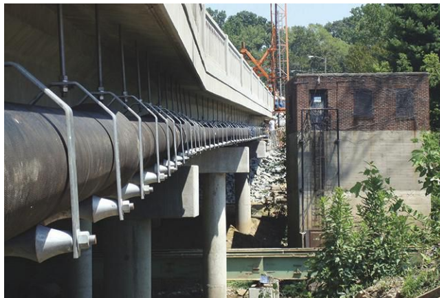
A ductile iron-forced water main was placed beneath this bridge.
