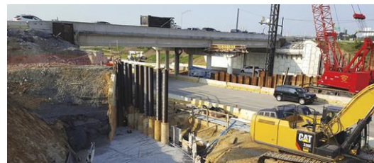
A shored MSE wall stabilized the bridge.
