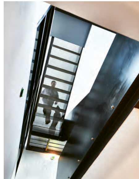
This page: The perforated-steel, switchback stair permits light to pass through to the ground level from a series of skylights above. Although the result is tidy, careful surgery was required to marry new structure to existing beams and to shore up weak areas.
