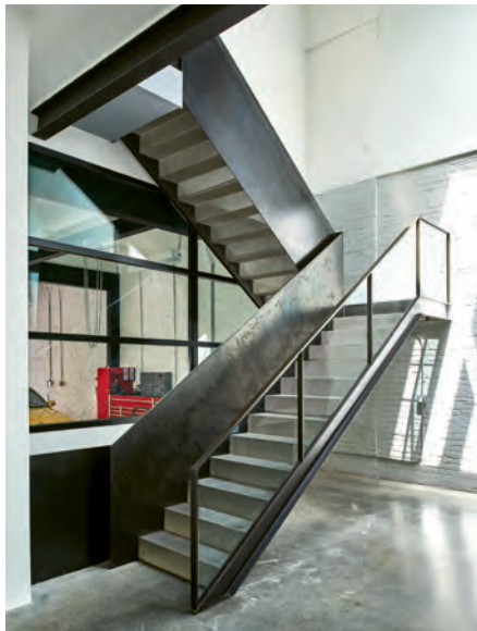
This page: The perforated-steel, switchback stair permits light to pass through to the ground level from a series of skylights above. Although the result is tidy, careful surgery was required to marry new structure to existing beams and to shore up weak areas.
