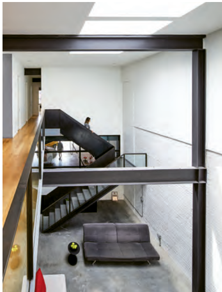
This page: The perforated-steel, switchback stair permits light to pass through to the ground level from a series of skylights above. Although the result is tidy, careful surgery was required to marry new structure to existing beams and to shore up weak areas.
