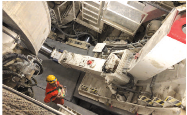
STEADY PROGRESS Inside the TBM, a worker guides a precast concrete lining segment into place. Caverns and tunnel interchanges (right) provide much-needed logistical space along the 55-km worksite.
