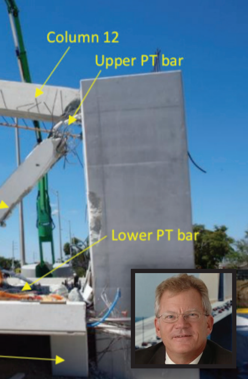
CRITICAL NODE Engineer Denney Pate stamped plans for pedestrian bridge where report claims key node at diagonal 11 was underdesigned.
