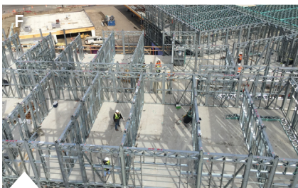
Prescient's 5D "Digital Thread" program guides A) laser drilling, B) robotic welding, C) QR coding, D) storage of finished panels at a 10-acre site in Colorado, E) trucking to the project, and F) installation at the site.
