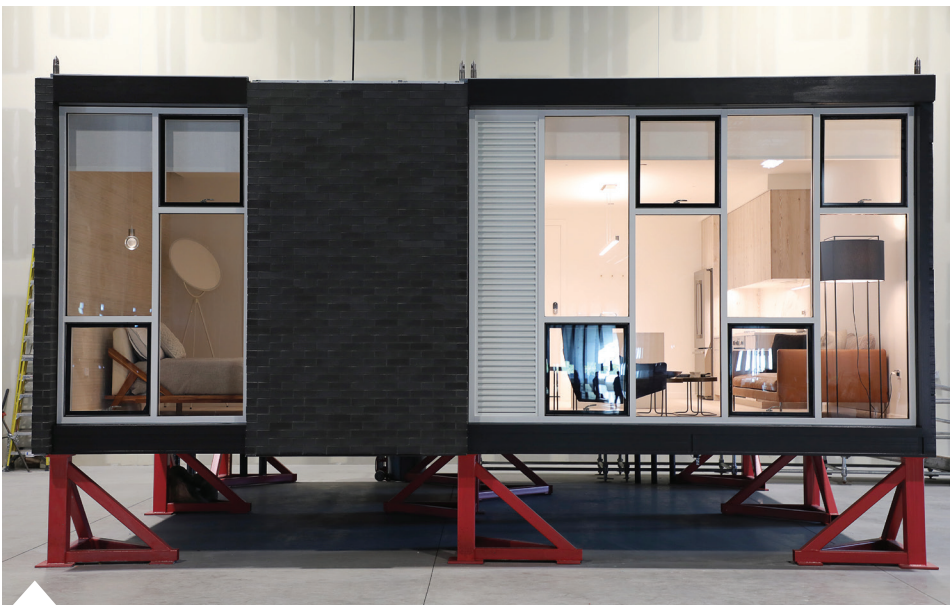
A “smart” apartment prototype on display in Skender’s Chicago factory. The steel-frame module uses the Z Modular/VectorBloc, a Lego-like steel connection system that “pins” the modules together. Factory production will allow assemblies to be held to a tolerance of \frac{1}{16} inch, says Skender’s Pete Murray.
