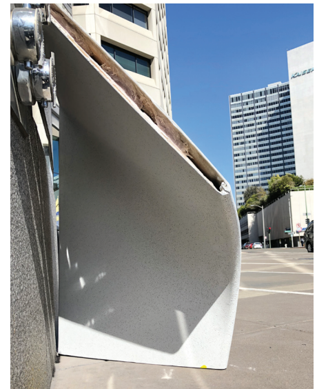
FIGURE 7. Partial, full-scale mockup showing hollow core cross-section
