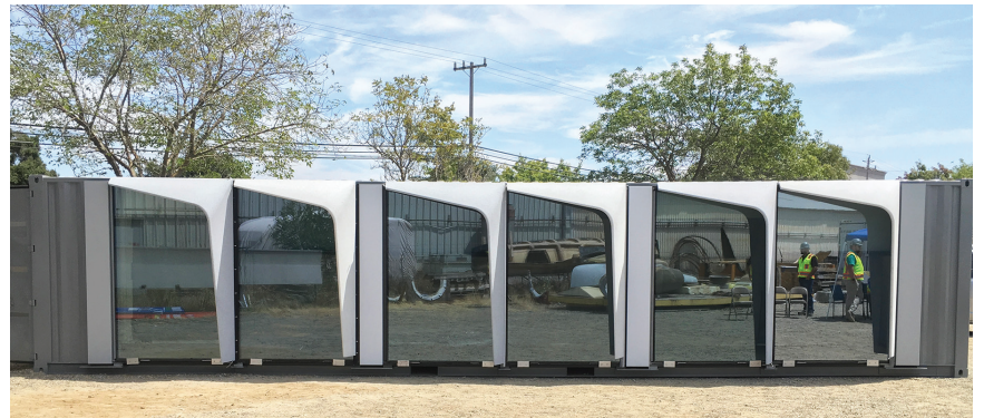
Physical mock-up of custom-shaped sunshades for 633 Folsom in San Francisco.
