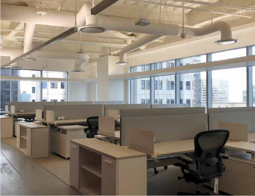
Arup’s new Los Angeles offices integrate daylight and electric illumination by means of an interior light shelf. The device shields the interior from glare and directs sunlight to the ceiling, thereby getting daylight farther into the interior. It incorporates tunable-white LEDs for times when natural light is not sufficient.
