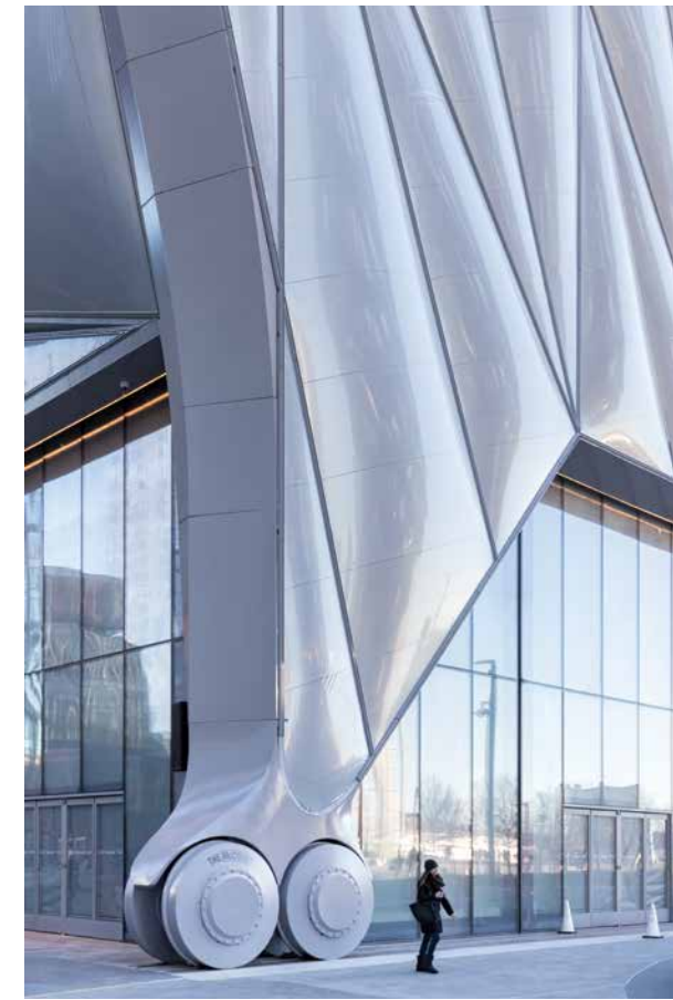
ROCK AND ROLL The building's retractable shell slides out on eight 6-foot-diameter bogie wheels (above).
