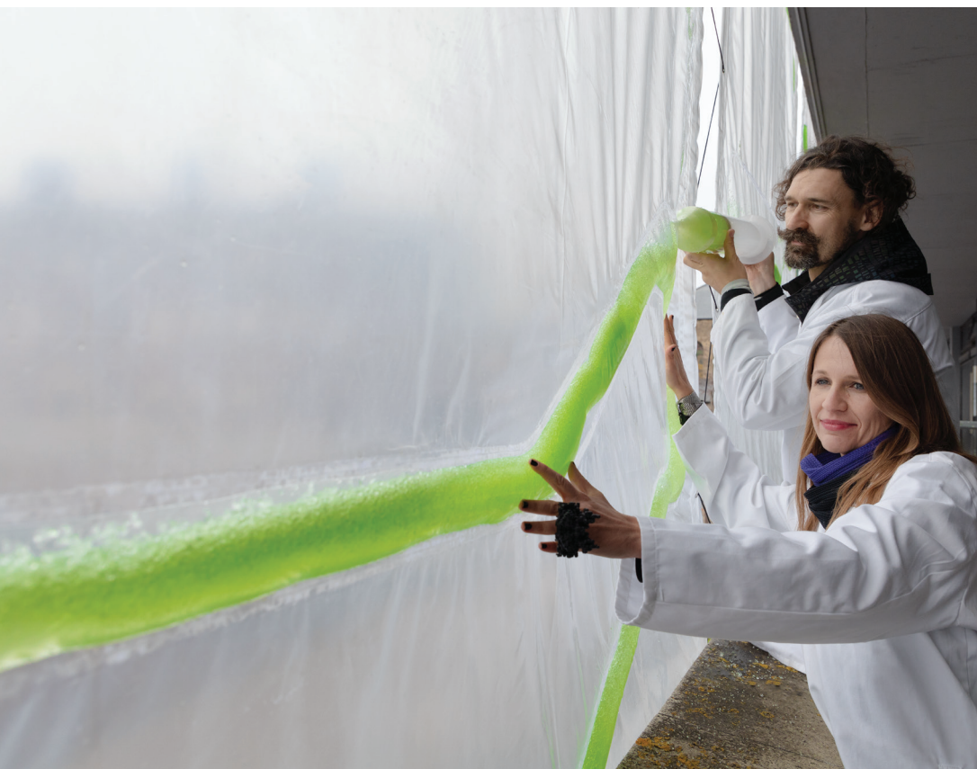
A membrane that integrates algae (above) and can be configured to provide shading while improving urban air quality has been developed by ecoLogicStudio. The system appeared on a facade in Dublin during a 2018 climate innovation summit (right).
