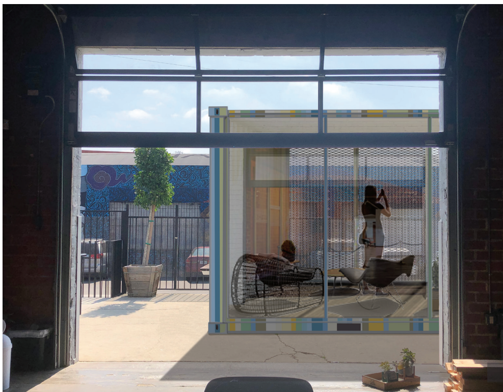
DO|SU Studio's InVert insulated glazing units incorporate leaf-like pieces of thermobiometal (above). As the pieces heat up in the sun, they toggle to provide shade. Even in shading mode (left), visibility to the exterior is maintained.
